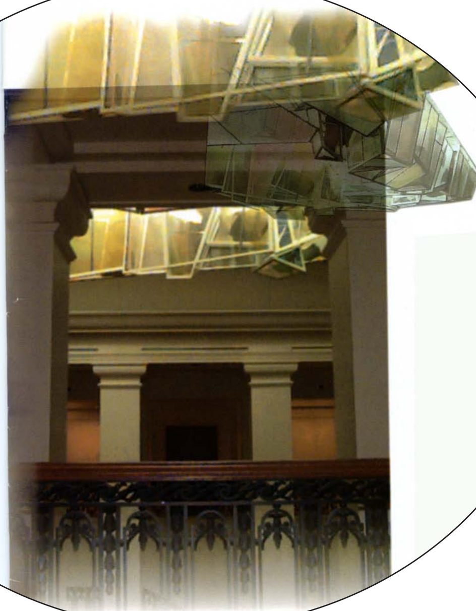
The “Falling Water Skylight,” formed from more than 500 pieces of glass, graces the Grand Hall of the Minnesota Judicial Center. 3M™ Scotchshield™ High Performance Safety and Security Film covers each piece of glass, ensuring the safety of viewers while retaining the beauty of the Skylight.
